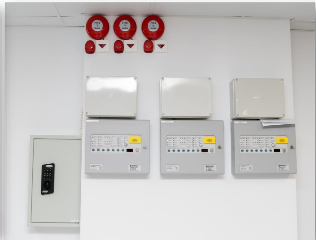
FIRE MONITORING AND CONTROL SYSTEM
