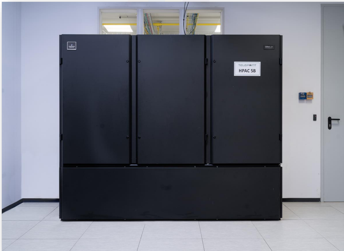
REDUNDANT CLIMATE CONTROL EQUIPMENT (N+1) - VERTIV
